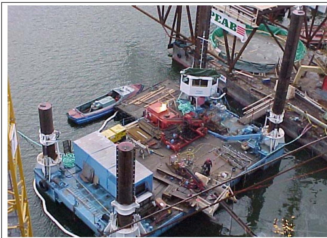
The use of a jack-up platform permits work to be carried out in similar conditions to those on land, specific benefits when using a jack-up platform compared to more traditional methods are: speed of operation, elimination/reduced downtime due to adverse weather, better quality of work for example drilling works, improved working and safety conditions and minimum interference to other marine traffic.
